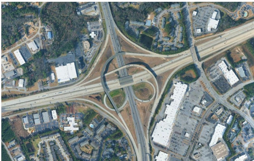
Interstate 20 at Interstate 520/Bobby Jones Expressway (Augusta-Richmond County)
