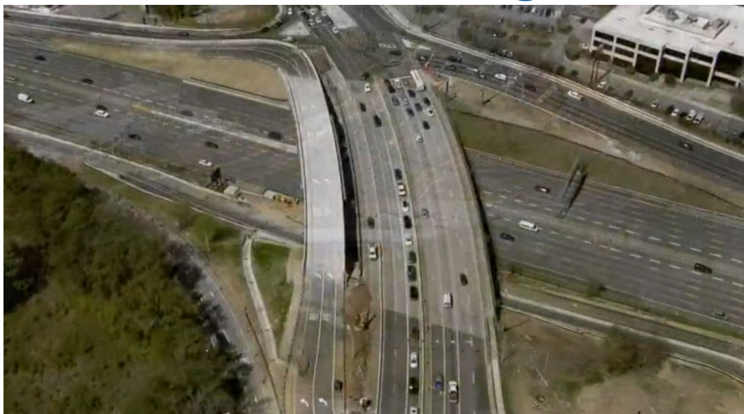
S.R. 42/North Druid Hills over Interstate 85 (DeKalb County)
